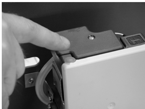
Fig. 22: Burner reset button
