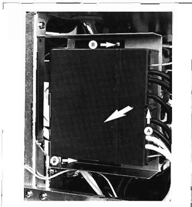
**5.7 To remove flue fan and venturi device**
