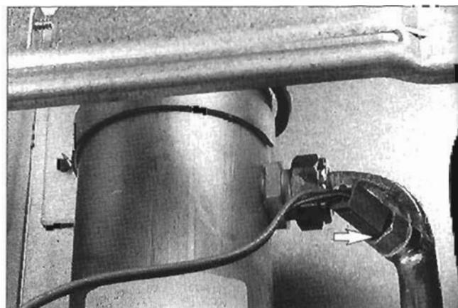
**5.18** To remove NTC probe on main circuit
