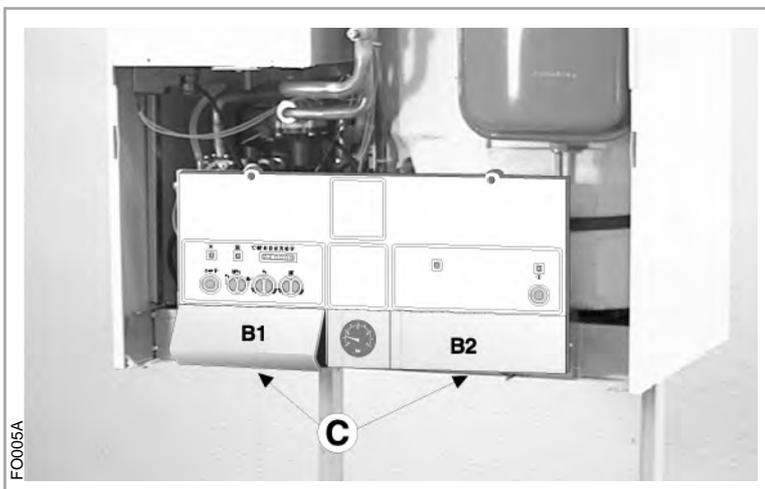
The boiler was designed to make regulation easy. To access the adjustment and control area, simply remove the cover by unscrewing the screws "A" and "C" and lift up the small service panels "B1" and "B2" respectively.
